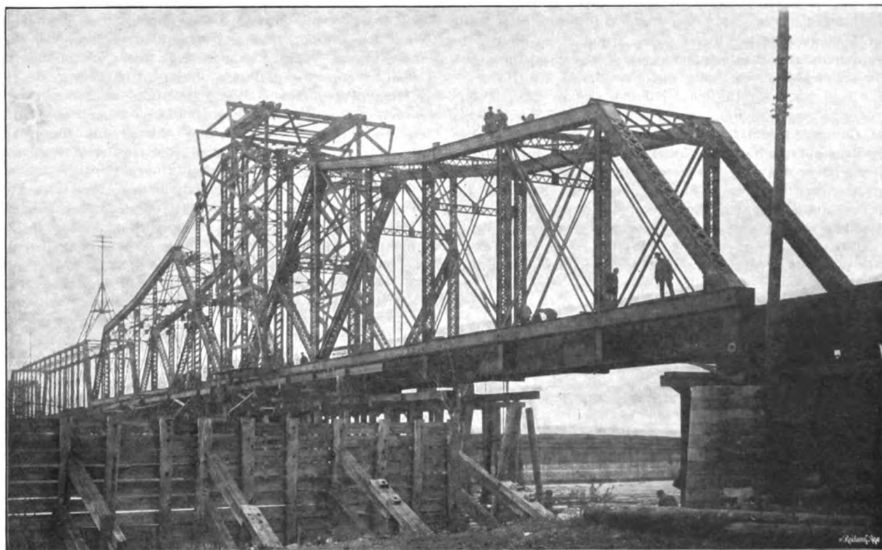
LACROSSE BRIDGE RENEWAL—DRAW SPAN OVER MAIN CHANNEL.
